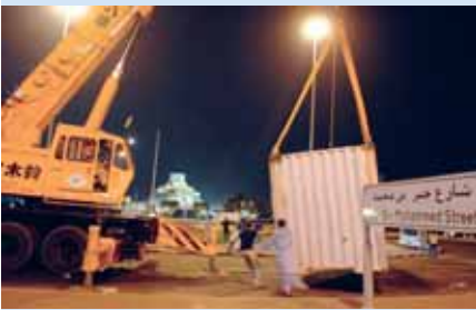
A crane helps clear the accident site after a trailer with a container tipped over at a roundabout near the Museum of Islamic Art yesterday.
